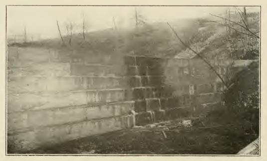
Fig. 2. Indiana University dam, seen from the valley below the dam. Each ledge is 4 feet high. Three ledges are concealed beneath the ground.
