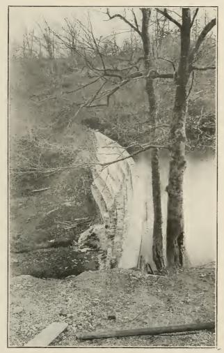
Fig. 3. Indiana University water-works dam from above north end, showing arching up-stream.
