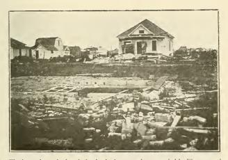
Fig. 10. The house from the foundation in the foreground was carried bodily across the street and then dropped to the earth and broken to bits. Wreckage may be seen in front of cottage on the right.
