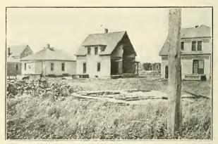
Fig. 4. House with end blown outward.
