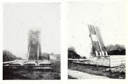
Fig. 2. (a) Down stream view of two Chanoine Wickets as they would appear in Dani No. 37. Shows the "props," their attachment and that of the timbers to the "horses" and the grooves that guide the "props" when the wickets are being raised or lowered.
