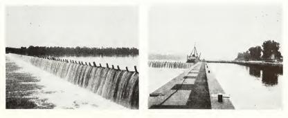
Fig 1. (a) Dam No. 49 located  $2\frac{1}{2}$  miles below Union Town, Ky. The "needles" are all in place helping to maintain full pool stage during the drought of 1930.
