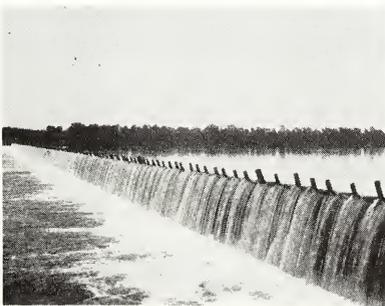
Fig 1. (a) Dam No. 49 located 2½ miles below Union Town, Ky. The "needles" are all in place helping to maintain full pool level during the drought of 1930.
