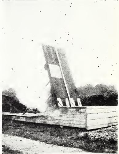
Fig. 2. (a) Down stream view of two Chanoiné Wickets as they would appear in Dam No. 37. Shows the "props," their attachment and that of the timbers to the "horses" and the grooves that guide the "props" when the wickets are being raised or lowered.
