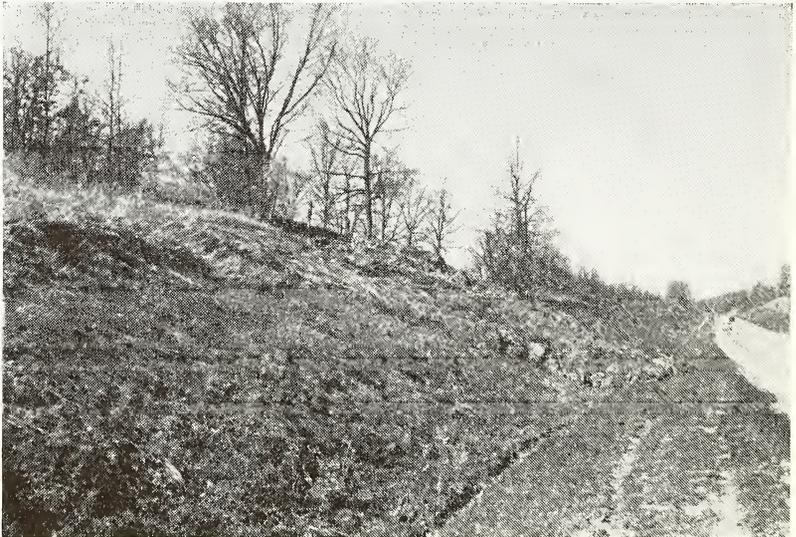
Figure 3. Mudflow on road cut in weathered Illinoian till along State Road 37 near Morgan-Monroe county line. The high clay content of the weathered till prevented it from remaining stable at the original cut dimensions, although a similar cut in unweathered till probably would have remained stable at that slope.
