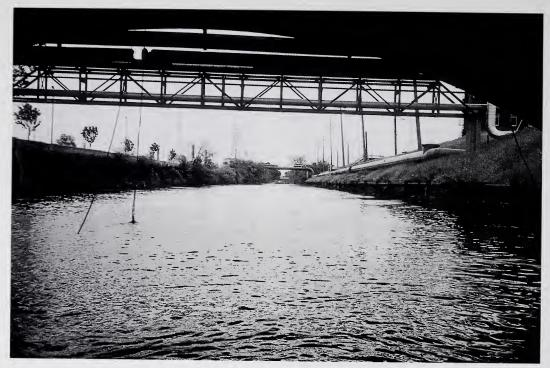
In addition to transportation crossings, the areas around the Grand Calumet River are heavily used by industry. Pipelines run along much of its length and across the channel. The banks have been heavily modified in order to maintain industrial equipment.
