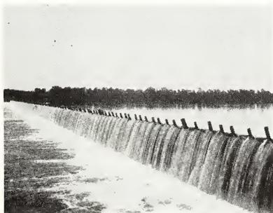
Fig 1. (a) Dam No. 49 located 2½ miles below Union Town, Ky. The "needles" are all in place helping to maintain full pool stage during the drought of 1930.
