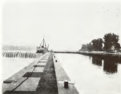
(b) The lock and a portion of Dam No. 49 and the tender boat. The lock has been filled ready to receive boats from up stream.
